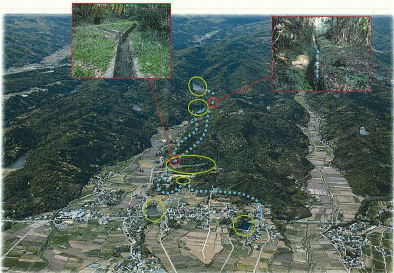
Multiple Interlinked Irrigation Pond System at Tsunai
